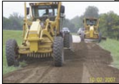
Gravel being spread by Levee Board crew.
