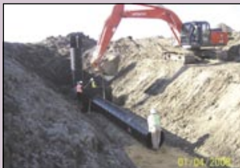
Phase II Construction - Installation of riser pipe.
