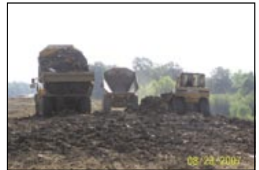
Topping Out Levee
