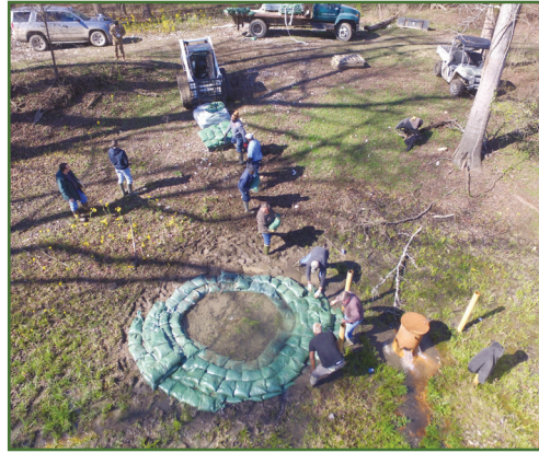
Crew Building Sandbag Ring Around Sandboil at Buck Chute (Feb. 27, 2020)
