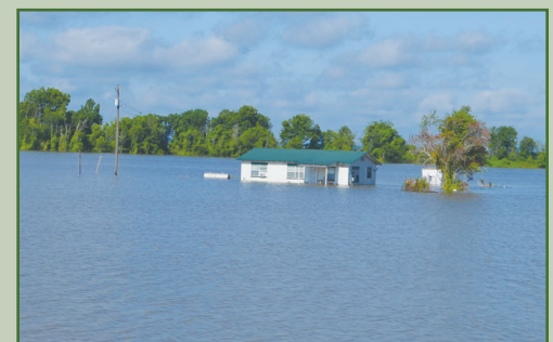
Flooded Home on Hwy 61
