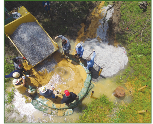
Crew & Corps placing Filter over Sandboil at Buck Chute (April 14, 2020)
