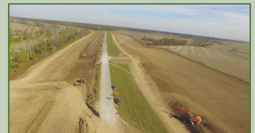
Item 462L – Aerial view of Berm and Levee Construction
