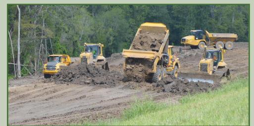
Item 465L – Placing Material on Riverside Embankment
