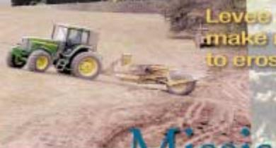
Levee Board crew and equipment make repairs to the levee slope due to erosions caused by ruts.
