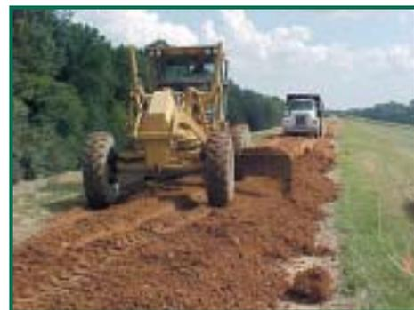
Levee Board Crews spreading Gravel
