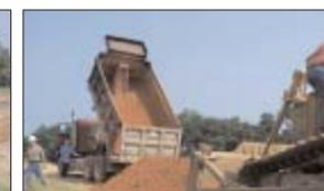
Item 477L - placing gravel on completed portion of levee
