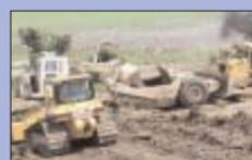
Bulldozers and scrapers remove slide soil material
