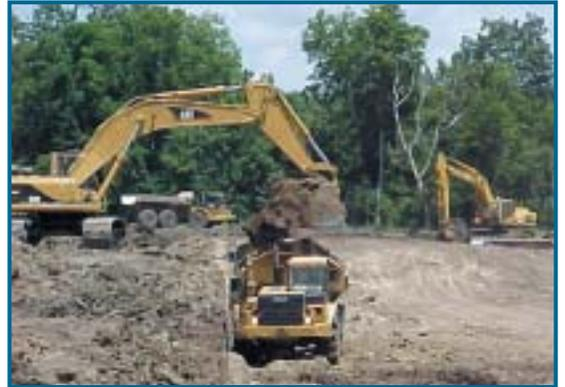
**Item 477L** - The Notice to Proceed was granted to ASA Enterprises of Jackson, MO on August 1, 2002. This is a 5.1 mile conventional levee enlargement project. Relief Wells were installed in 1997, therefore a berm is not needed.
